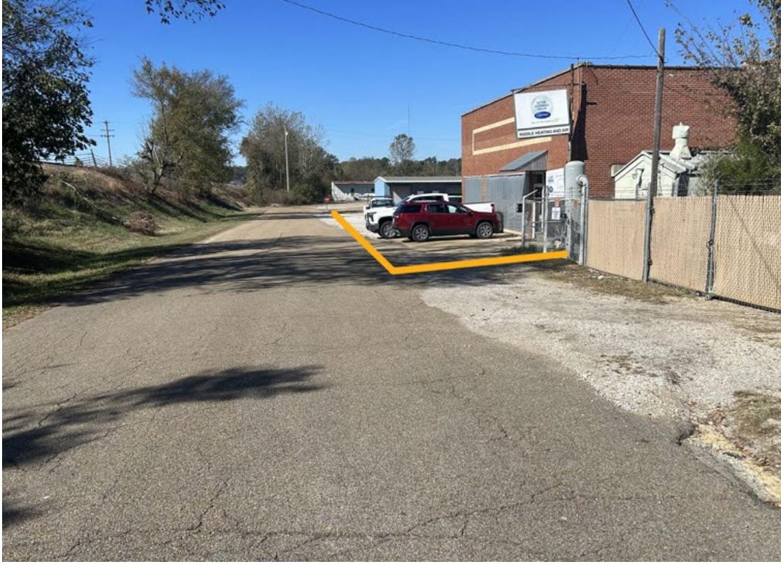
Photo 5. West end of APE along McGill Street, view facing west.
