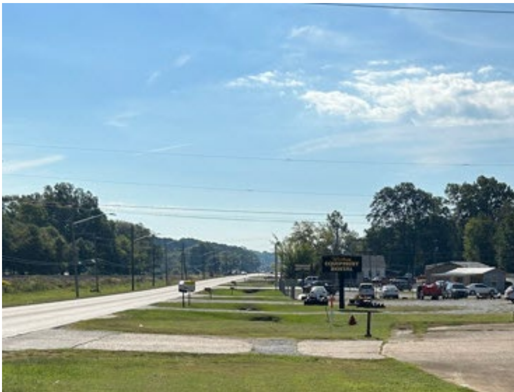
Photo 2. APE along W. Bankhead Street, view facing east.
